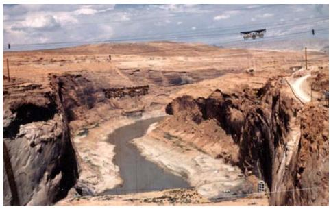
Before construction on the dam itself could begin, a coffer dam had to be built upstream from the site and diversion tunnels built around it. The work took a couple years. This photograph, from 1959, was taken from the new bridge that was also required to connect the two sides of the project. Note the cables traversing the canyon--materials were moved back and forth in this fashion. At the very bottom of the picture is the coffer dam.
