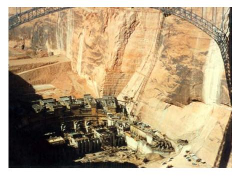
The new dam starts to take shape. By 1961, the bottom sections of the dam had been poured and the project moved quickly, despite a strike in 1961. By January 1963, the dam had been constructed to a sufficient height to close the diversion gates and to stop the river's flow.
